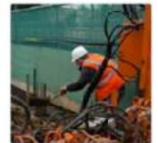
"construction worker in orange safety vest is working on road"
